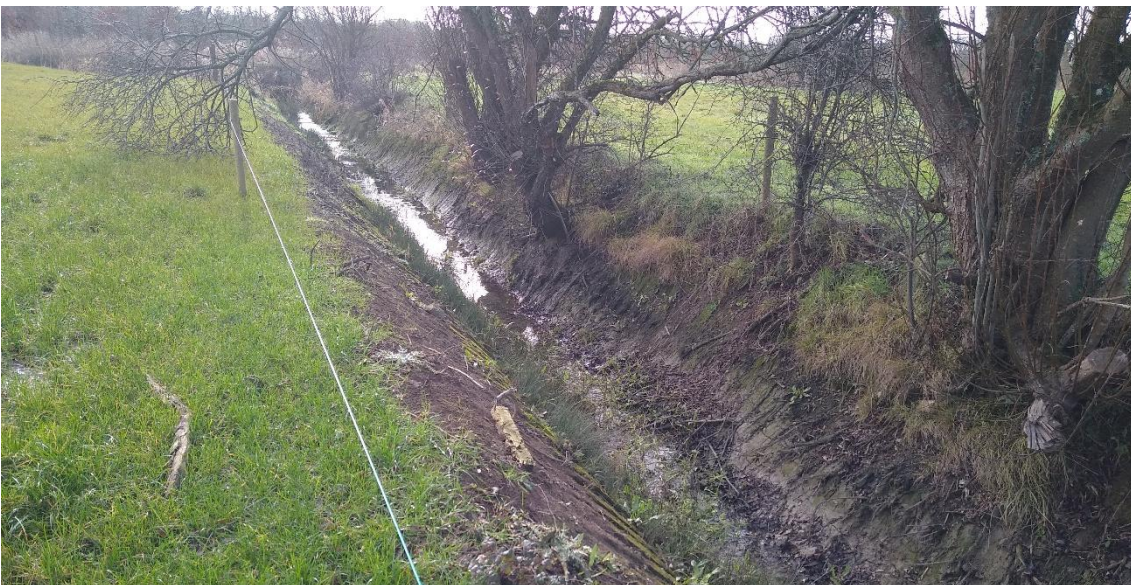
Figure 3-4: Drainage ditch (FW4). Note the presence standing water backfilling from the river
